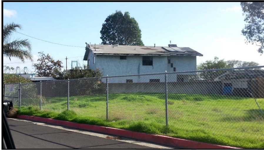
Figure 9. Photos of Knoll Hill Area (Site #5)
